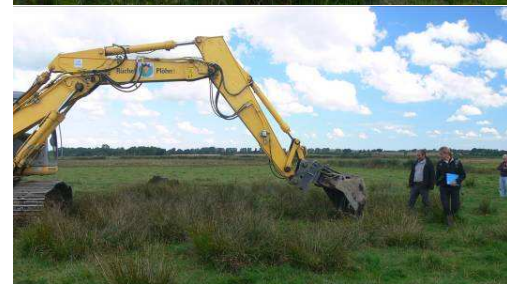
Test holes for restoration of depressions
